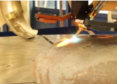
Cut radial and hill-side holes with weld preparations such as V and K bevels.
